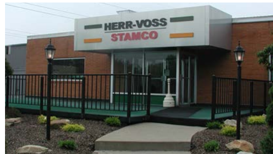
▲ Herr-Voss Stamco office building, USA
